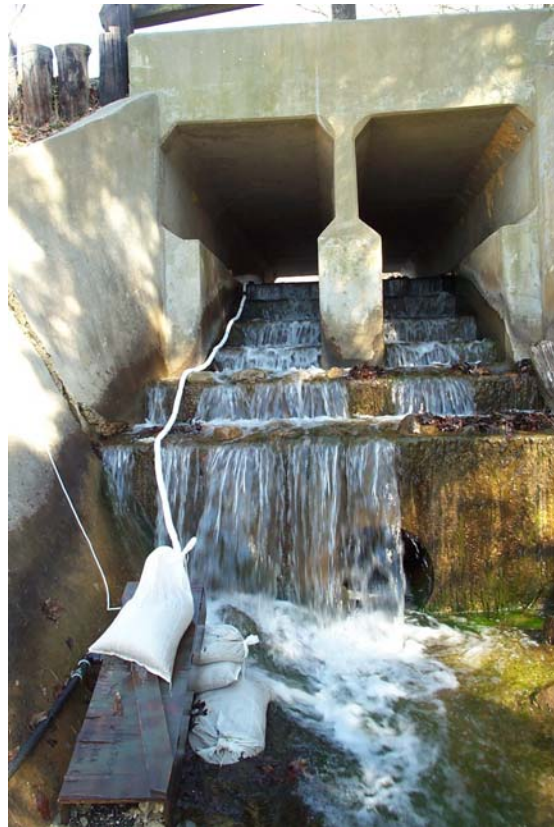
Figure 6. An Irish eel ramp showing its configuration. The arrows indicate the flow of water as well as eel movement.
