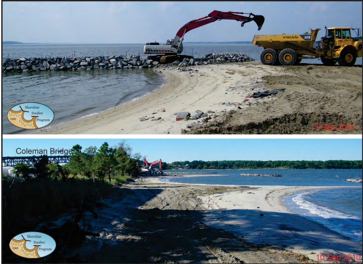
Figure 6-9. VIMS West shoreline during construction of the living shoreline in 2010. Photo credit: Shoreline Studies Program, VIMS.
