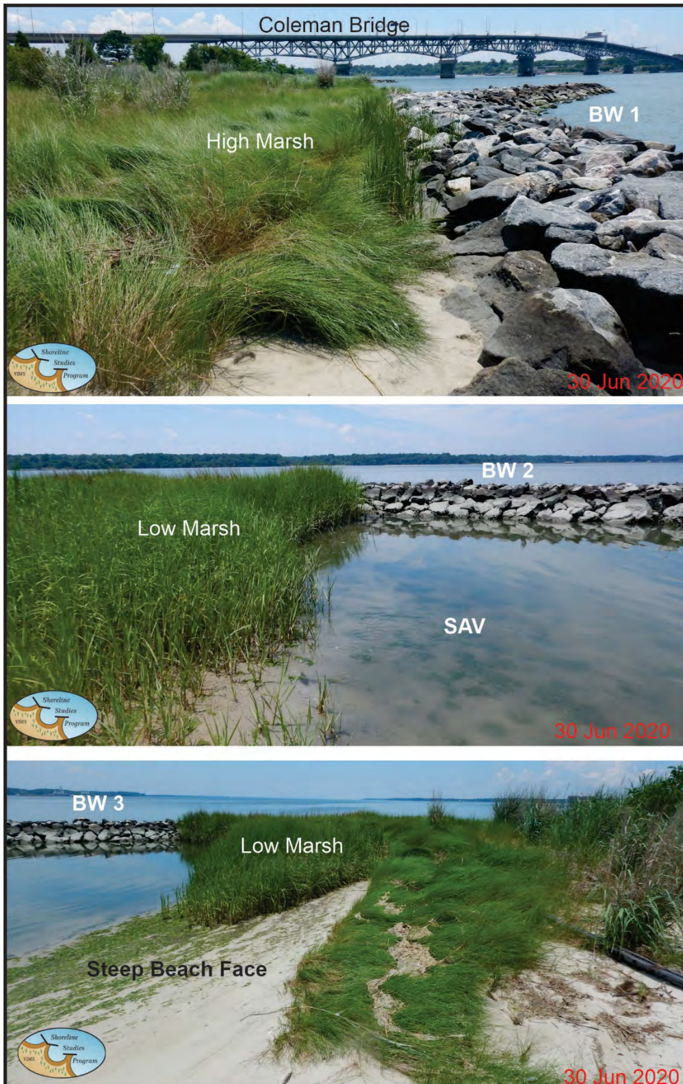
Figure 6-18. State of VIMS West in June 2020 about 9.5 years after construction. The structures are stable and the high and low marsh grasses are lush. SAV has colonized in the embayments. Photo credit: Shoreline Studies Program, VIMS.
