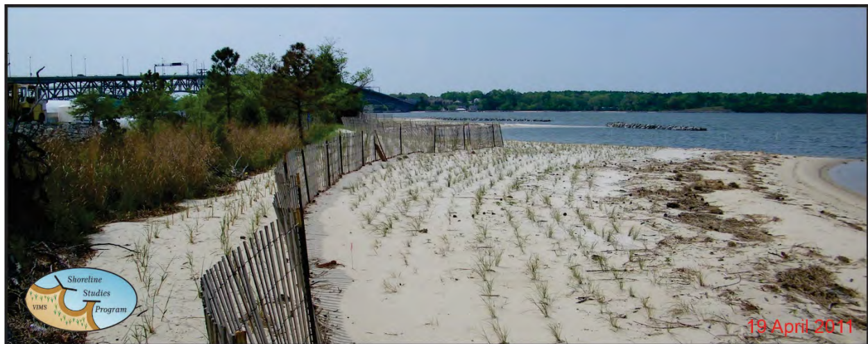
Figure 6-11. Planting of beach grasses took place the spring after construction. Photo credit: Shoreline Studies Program, VIMS
