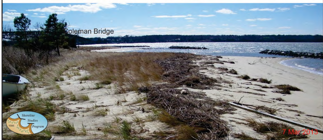
Figure 6-12. Photos taken at VIMS West during the passage of the March 2013 Northeast storm. Water levels are high enough to overtop the structures, but by the next day, tide levels had dropped. Photo credit: Shoreline Studies Program, VIMS
