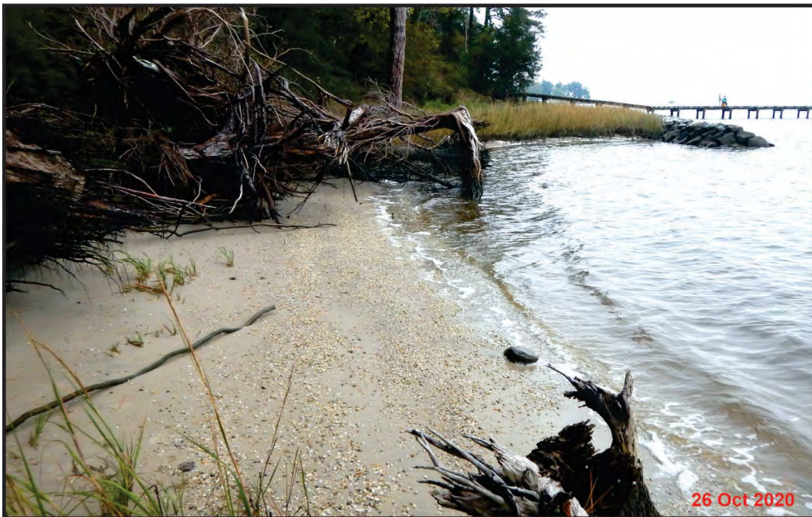
Figure 7-9. Eroding shoreline north of Sill 2. An additional structure is needed to protect the bank along this section of shoreline. Photo credit: Shoreline Studies Program, VIMS.
